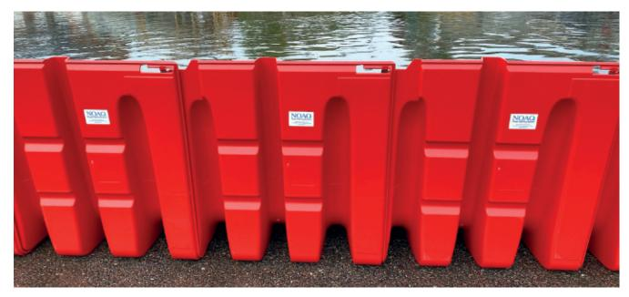
The NOAQ Boxwall is a freestanding temporary flood barrier. It is designed specifically for the urban environment, with even surfaces like asphalt streets, but it works as well on lawns etc.
